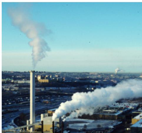
*Flue gas plumes from stacks with a height above and within an inversion layer, respectively.*
