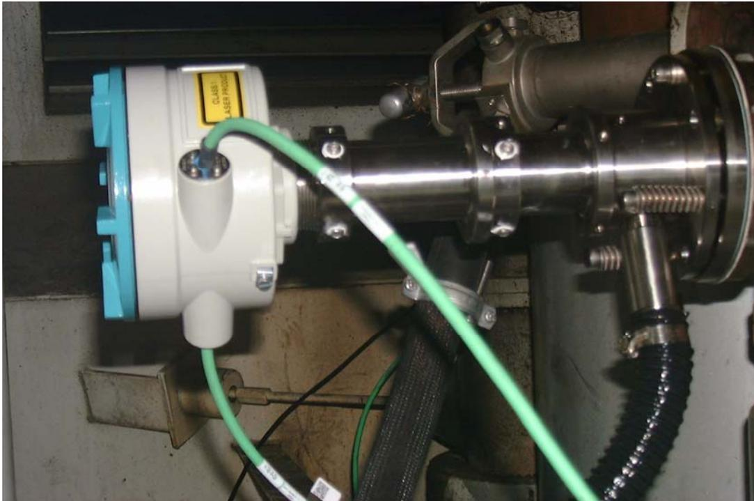
Figure 14. A picture of the LDS 6 transmitter mounted on the exhaust channel of a ship.
